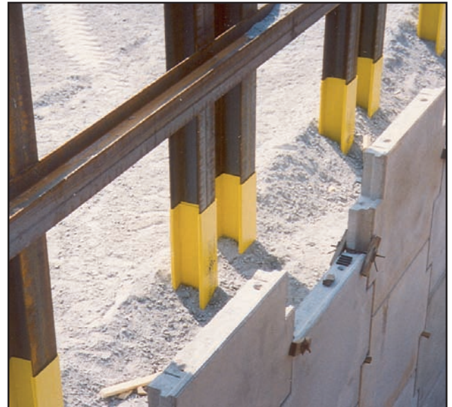
Yellow Jacket™ piles embedded behind an MSE wall bridge abutment.
