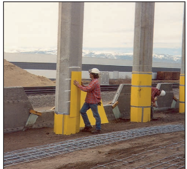
A simple, fast, economical friction reduction solution for pressed concrete pile shapes.
