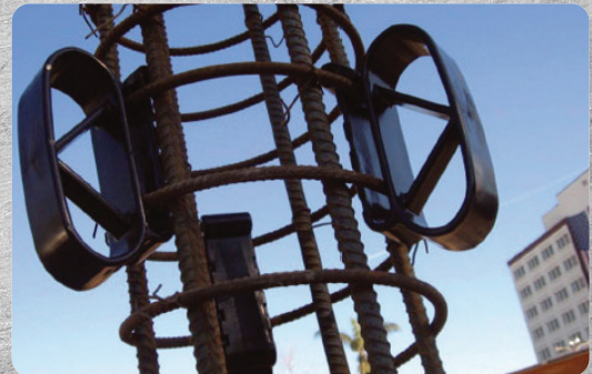
Cage clips attached at 3-points; ready for installation
