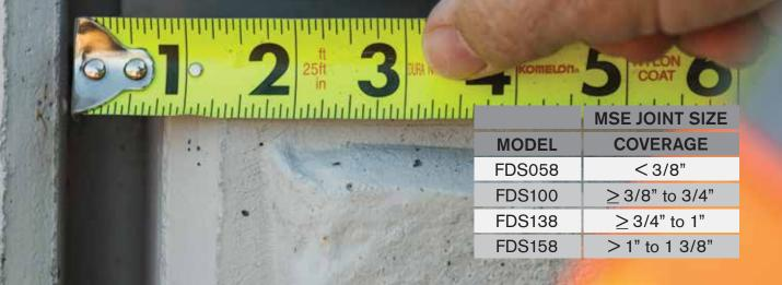
Insert FDS 1" into joint. FDS should be installed into the joint with the FDS seam facing towards the wall.
