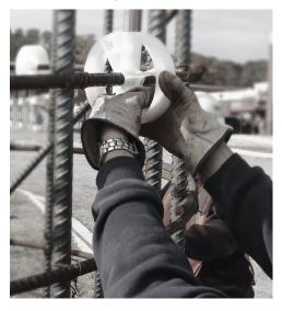
Guiding rebar cage into drilled shaft with ShaftSpacers attached
