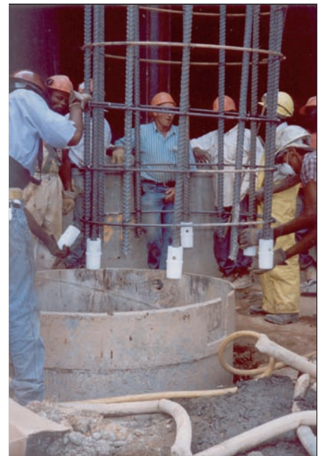
Fabricated rebar cage with Barboots ready for insertion into excavated shaft.
