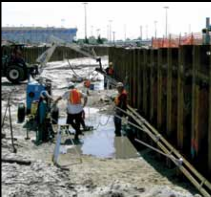
Tensioned Immediately Following Installation
