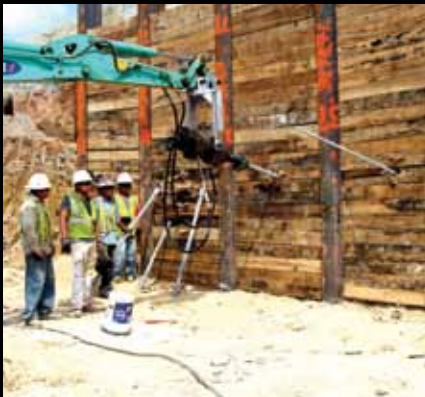
Soldier Pile & Lagging Shoring
