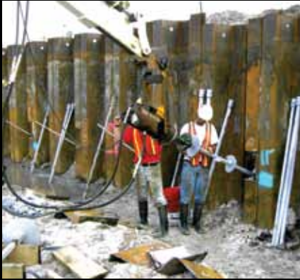
Sheet Piling Shoring
