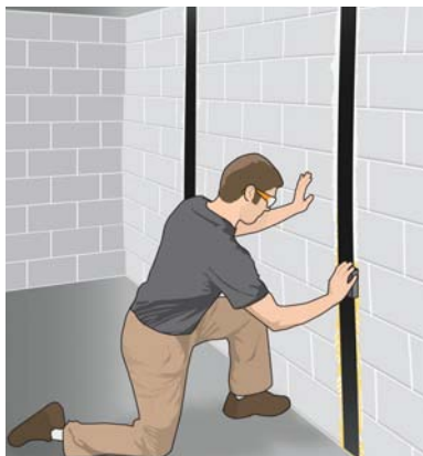
Step 3: Place StrongHold™ Carbon Strap to Wall
