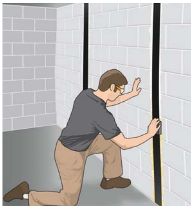
Step 3: Place StrongHold™ Carbon Strap to Wall
