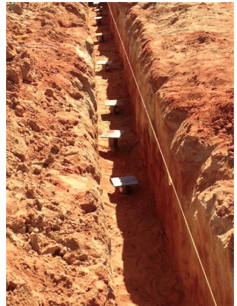
New Construction Plates installed to allow for pile and footing connection
