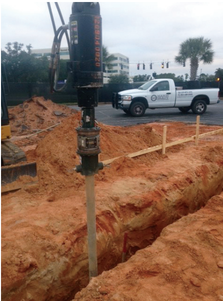
RS3500 Pipe Extension installation
