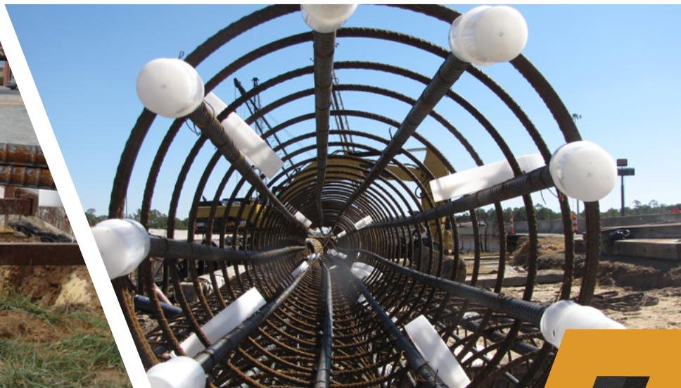
Rebar cage staged with Barboot supports attached
