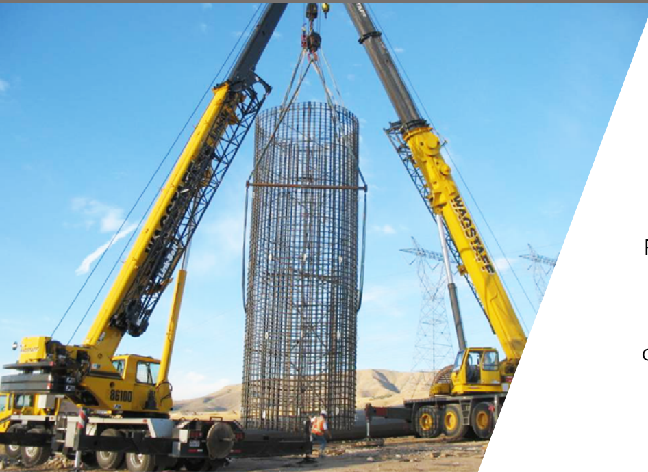
ShaftSpacers attached along large-diameter reinforcing cage
