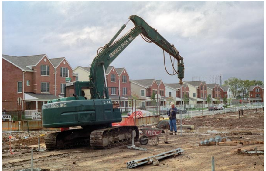
Phase II installation with completed Phase I homes in background
